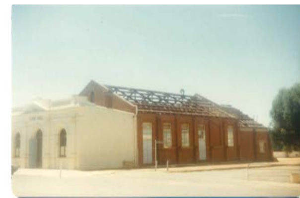
1984 Upgrade Works including new roof + ceilings + facade upgrade.
