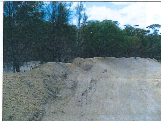
Images showing banked turn with uneven surfaces, vegetation in close proximity to track and evidence of tyre marks on higher aspects of turn. The close proximity of vegetation increases potential for impact to occur.
