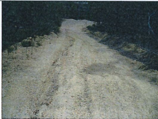
Images showing erosion wash outs on downhill section of the track which could increase potential for loss of control to occur.
