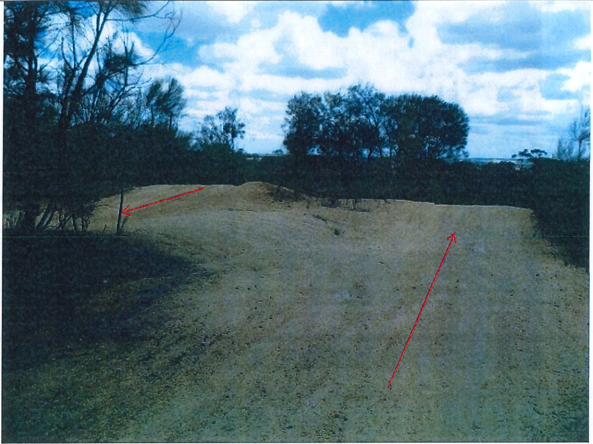
Image showing aspect of track where opposite directions of travel occur, increasing risk of collision should a rider cross over to the other track element especially as ground contours partially obscure vision.
