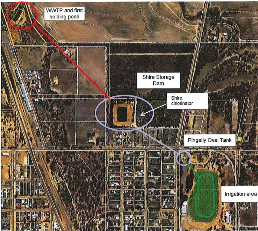
Wastewater transfer from WTP to Shire storage dam, storage tank and irrigation area
